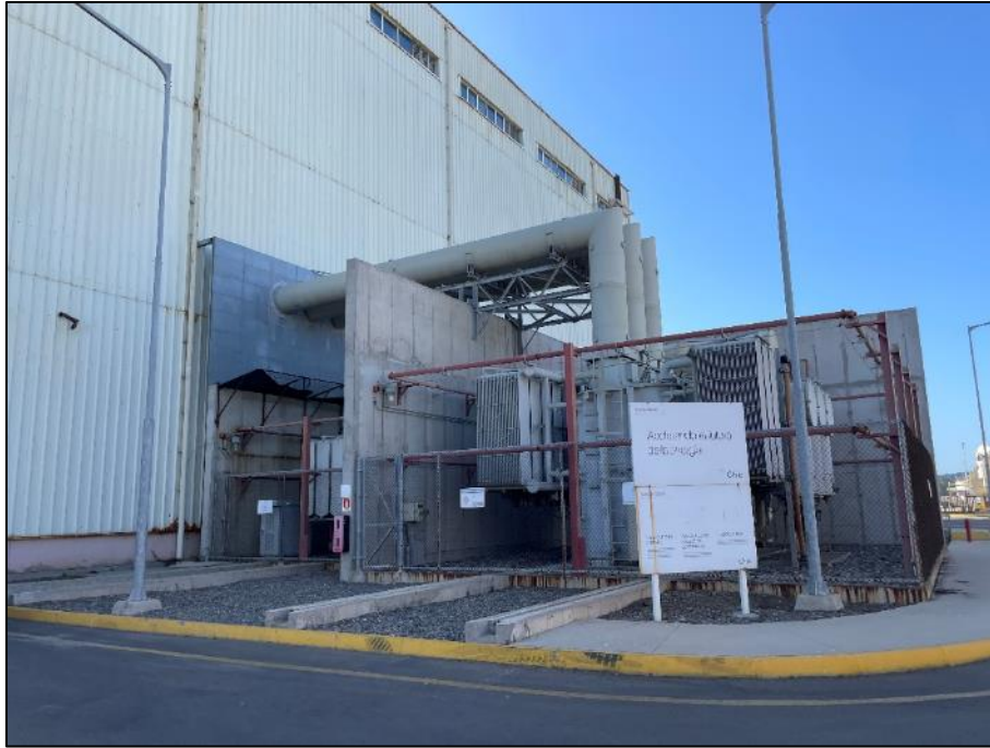
Unit V4 GSU Transformer (right) and Auxiliary Transformer (left)
