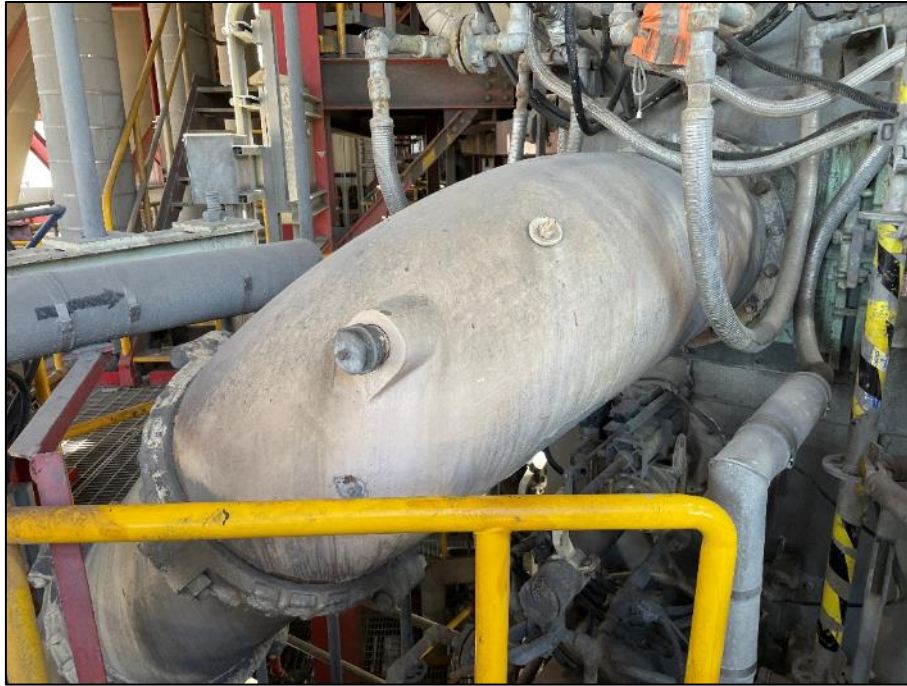
Elbow with Internal Wear Plate, Boiler Unit V3
