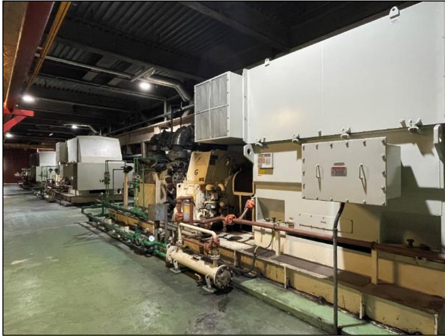
Cooling Water Recirculation Pumps, Unit V3
