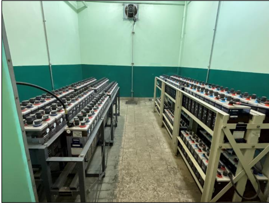
Battery Room with Forced Extraction and Hydrogen Sensor
