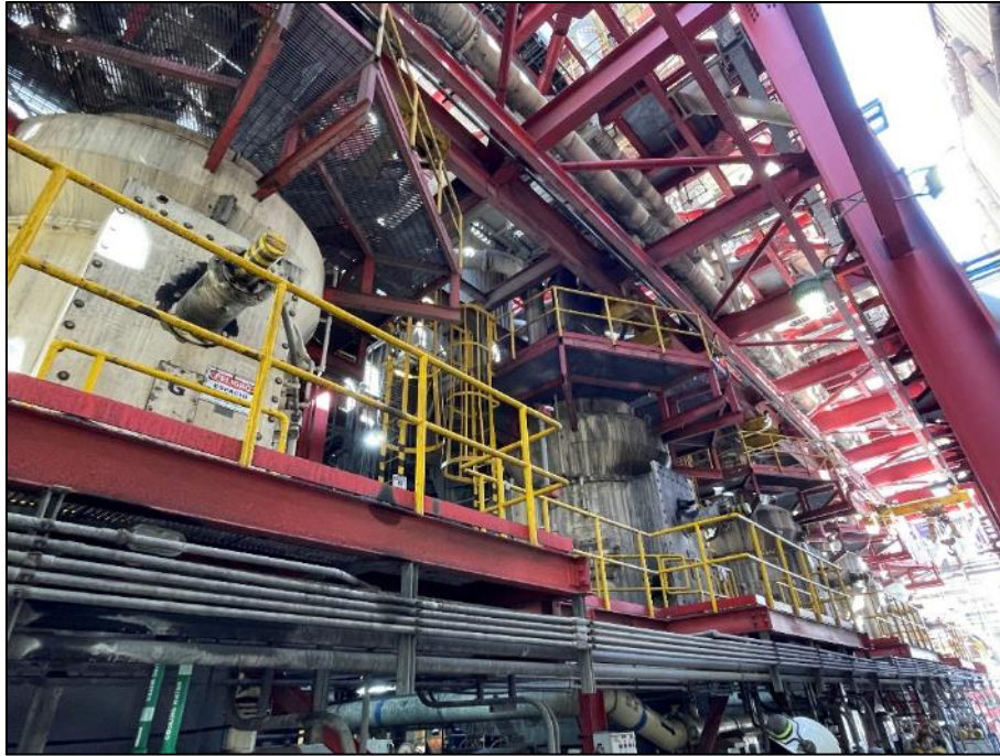
Coal Pulverizers, Unit V3
