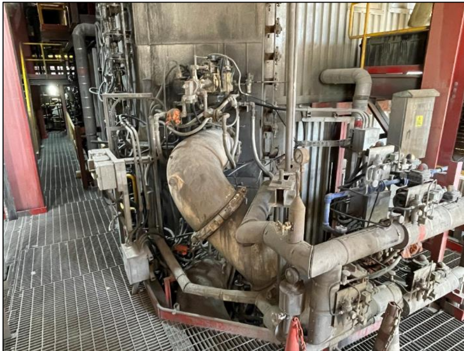
Fuel Injector for Boiler Startup, Unit V3
